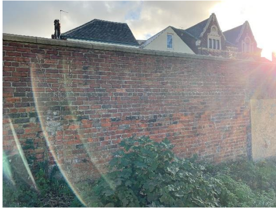
Photograph 21: Wall Section 4, Rebuilt at high level to the rear.
