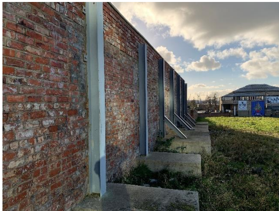
Photograph 23: Wall Section 4, restraint posts and infill masonry to windows.
