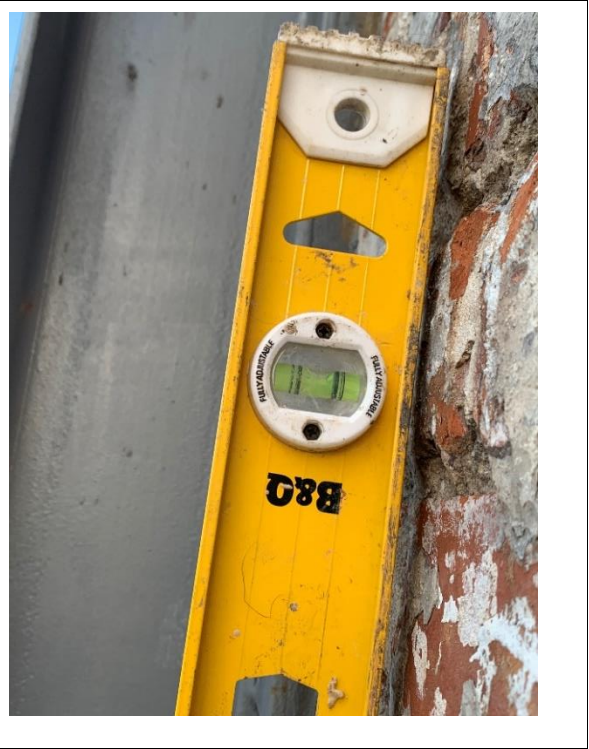
Photograph 30: Wall Section 3, spirit level used to check verticality.
