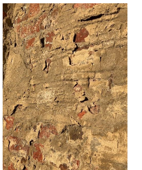
Photograph 36: Chimney West Elevation
