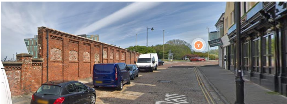
Figure 1: Façade to the former Staiths House now forms part of the boundary wall.
