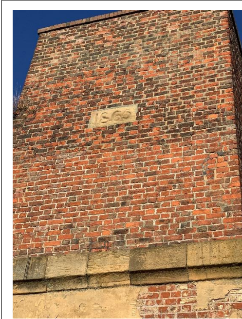
Photograph 33: Chimney West Elevation
