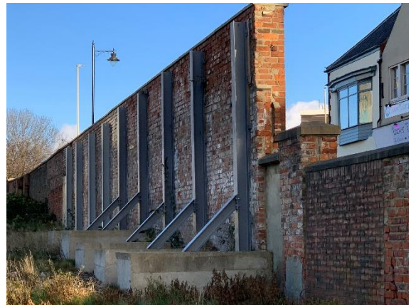
Photograph 24: Wall Section 4, restraint posts.
