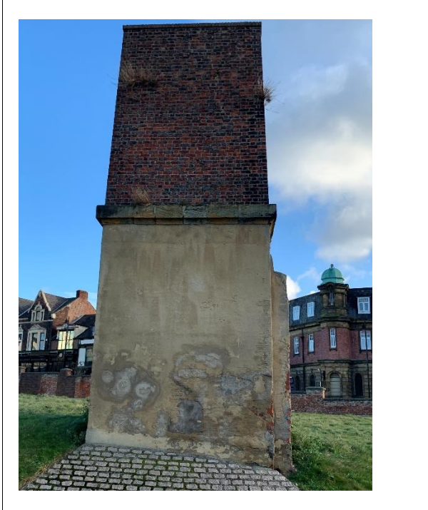
Photograph 31: Chimney North Elevation
