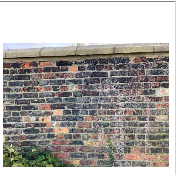
Photograph 20: Wall Section 4 rear.
