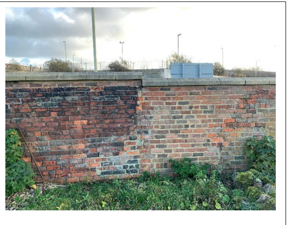
Photograph 18: Wall Section 4, Repair to rear of wall with different brickwork.
