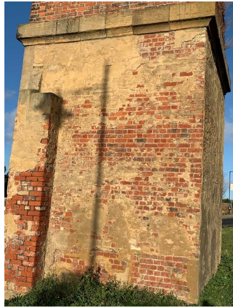
Photograph 34: Chimney West Elevation
