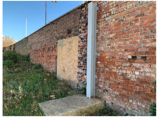
Photograph 22: Wall Section 3, restraint post to rear.
